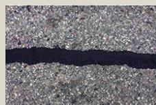
Sealed Crack
